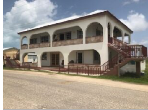
The New Barbuda Council Building, rebuilt with the help of UNDP funds
